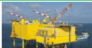
German Submarine Power Transmission Business for offshore wind power plants
