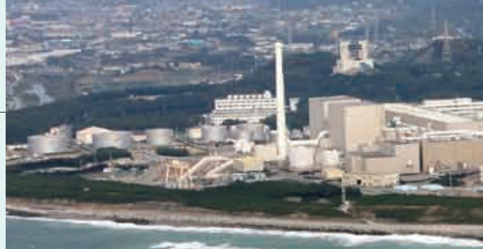
Hamaoka Nuclear Power Station
