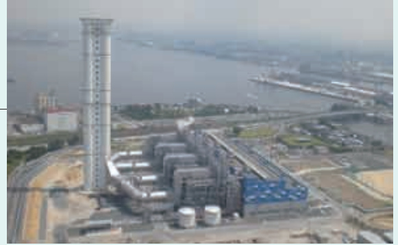
Shin-Nagoya Thermal Power Station Group No. 8
