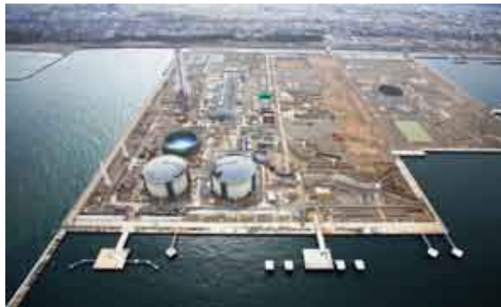
Joetsu Thermal Power Station (March 2010)
