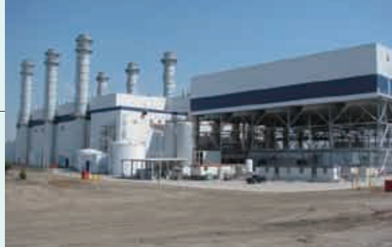
Goreway Power Plant, Canada
