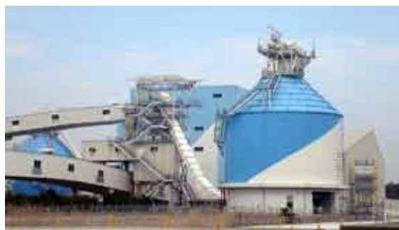
Biomass fuel facility (Hekinan Thermal Power Station)
