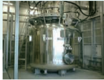
Superconducting Magnetic Energy Storage System (SMES)
