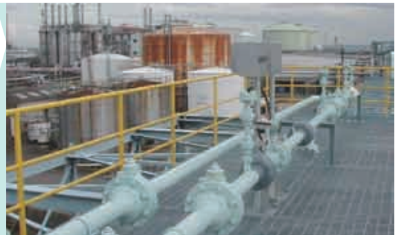
Gas supply facilities
