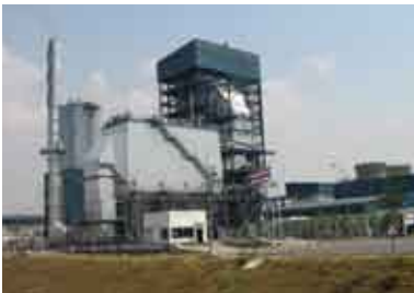
Rice Husk Power Station (North-central Thailand's Pichit Province)
