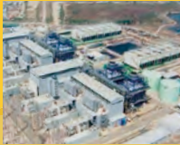
▲ Ratchaburi gas thermal IPP project in Thailand
