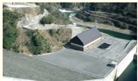
▲ Tokuyama Hydroelectric Power Station
