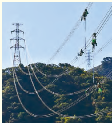
▲ Installing interphase spacers
