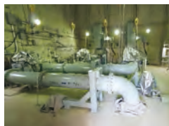
Emergency seawater intake system
