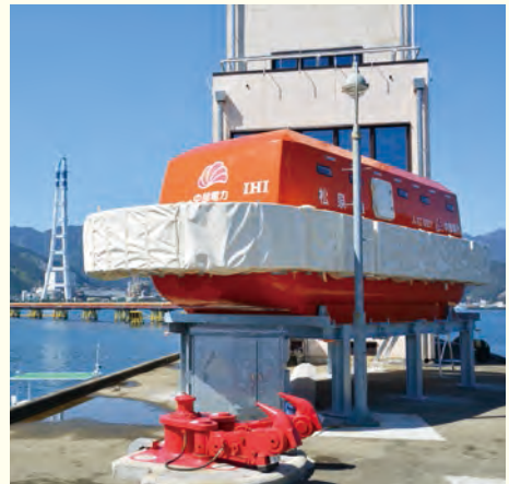
▲ Lifeboat installed at Owase-Mita Thermal Power Station
