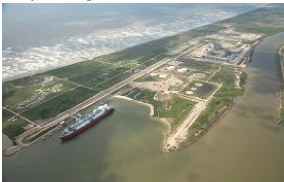
Existing Regasification Facility
