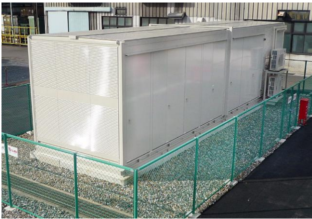
System for compensation of short-term power disruptions W 12.3 m × D 3.2 m × H 3.5 m 6,600 V, 1,000 kVA, 600 kW×11 sec compensation
