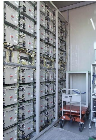
Lithium-ion capacitor banks
