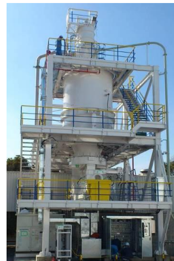
< Facility for receiving carbonized sewage sludge fuel >
