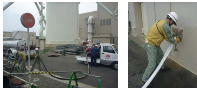
Check of viability of pumping water using portable power pumps
