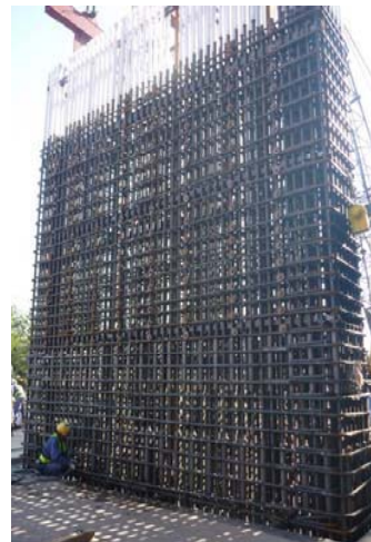
Reinforcing bar assembly installation
