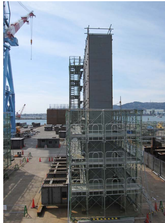
Cover shot of the wall section (floor slabs and vertical walls) temporarily assembled at the factory (February 28, 2012)
