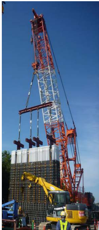
Reinforcing bar assembly installation
