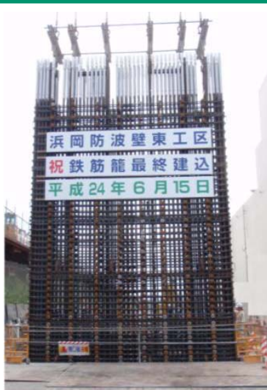
June 15, Final installation of breakwater foundation June 16, Concrete placing
