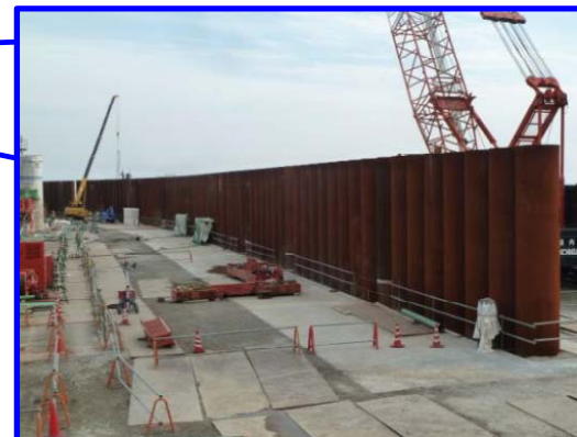
(Cover shot) After the driving work of steel pipe sheet piles
