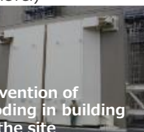
Prevention of flooding in building on the site Large equipment access way of building (Strengthening water tightness and pressure-resistance)
