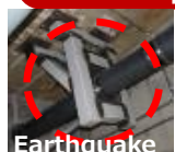
Earthquake Work to reinforce supports for pipes
