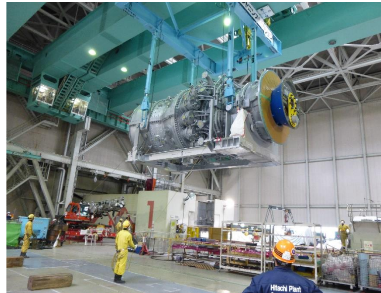
Installing a newer gas turbine
