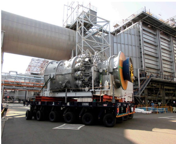
Carrying a gas turbine on the premises
