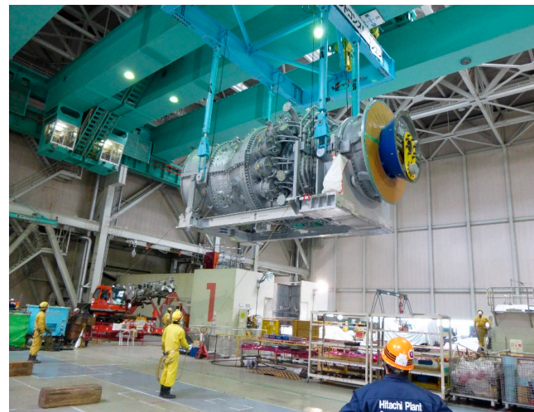
Installing a newer gas turbine
