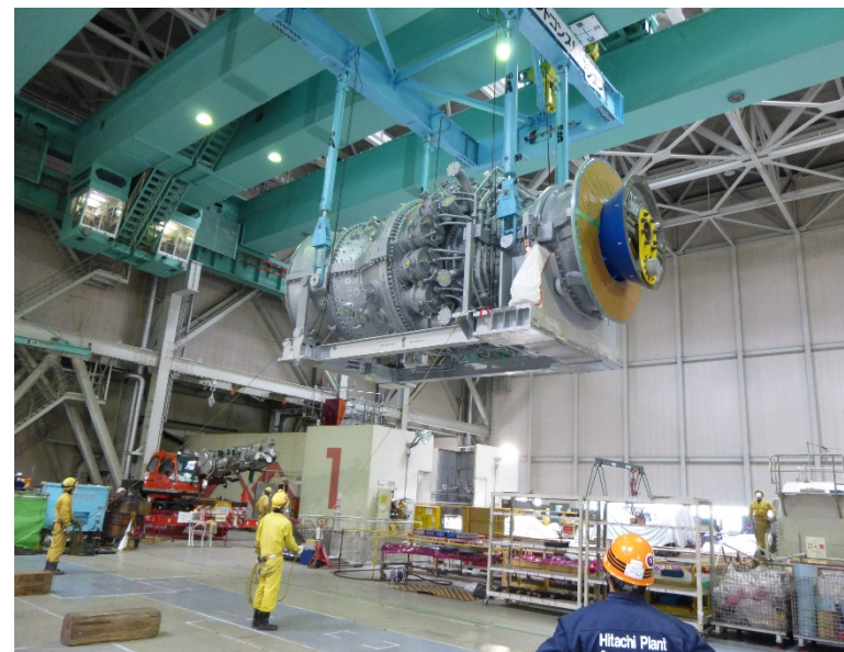
Installing a newer gas turbine
