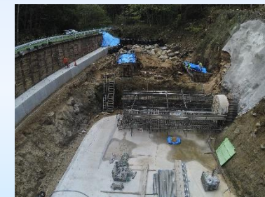
The situation of the construction of Ogurogawa dam of Seinaiji Hydroelectric Power Station
