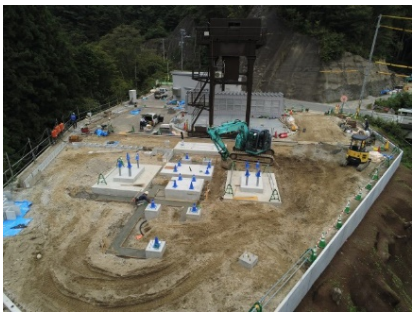
Seinaiji hydro (current status)
