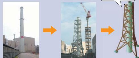
Construct a steel support tower to support the exhaust pipe of approximately 100 meters in height.
