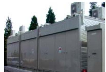
Uninterruptible power supply system incorporating a high-voltage, high-capacity double layer capacitor
