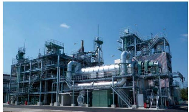
Sewage-sludge-to-fuel conversion facility in Kinuura East Purification Center
