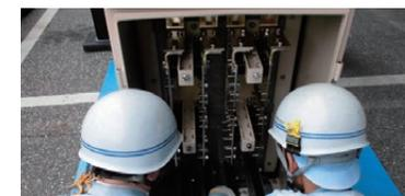
Removal of transformer tower doors (work done simultaneously)
