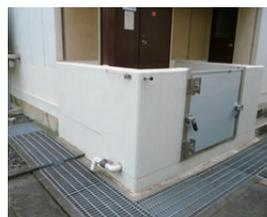
Tsunami protection measures of substation buildings (floodwall equipment)
