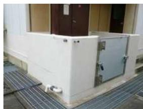
Tsunami protection measures of substation buildings (floodwall equipment)
