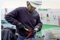
Service drop line dismantling work
