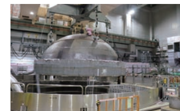
Scene of the removal of the reactor pressure vessel upper head
