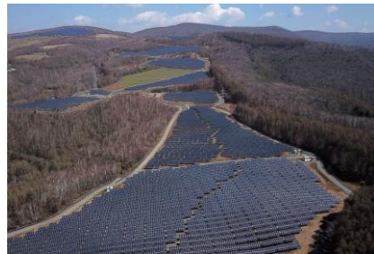
Miyako Kuzakai Solar Park
