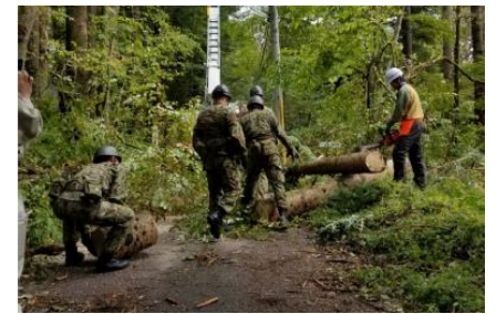
Trimming and culling of trees in collaboration with Ground Self-Defense Force
