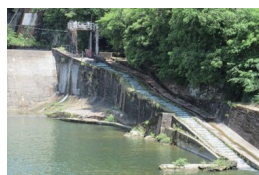
Fishway installed in a dam
