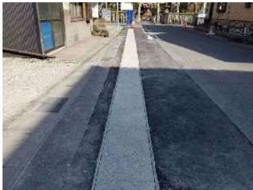
復旧完了 (As 舗装)
