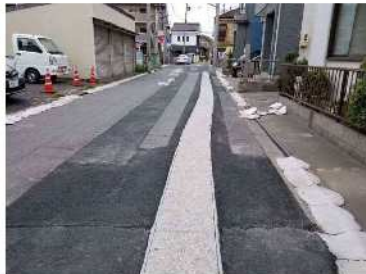
据付完了 (As 舗装) (曲線部施工状況)
