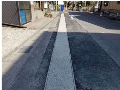
復旧完了 (As 舗装)
