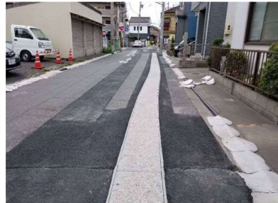
据付完了 (As 舗装) (曲線部施工状況)
