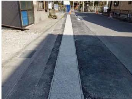
復旧完了 (As 舗装)
