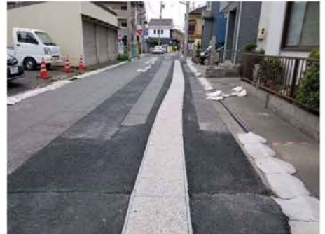
据付完了 (As 舗装) (曲線部施工状況)
