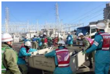
Installation work for connection cables
