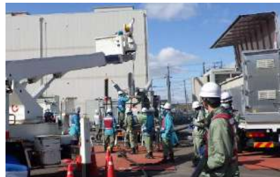
Work for connecting cables to mobile substation
