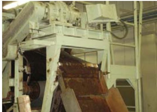
Compactor squeezes out sludge at the treatment facility
