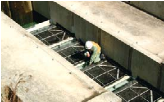
Purification facility using Circulash for wastewater containing lead at local government target range
