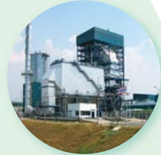
Rice Husk Biomass Power Generation Project in Thailand
