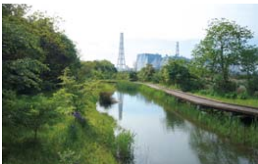
Circulating waterway (pond) at the Hekinan Thermal Power Station
