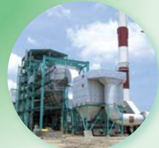
Oil Palm Empty Fruit Bunch Biomass Power Generation Project in Malaysia
