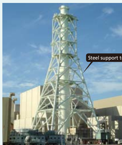
Construction to improve seismic tolerance: Renovation work on the exhaust stack for Unit No. 4 included construction of a steel supporting tower.
