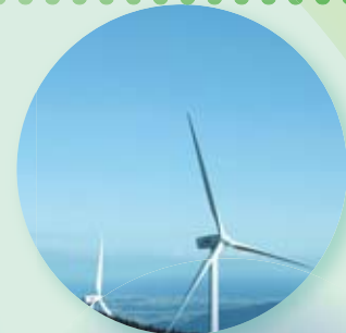
Wind power generation business
