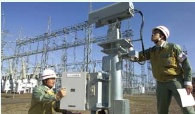
Substation observation and inspection work
