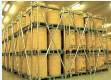
The drum cans stacked on the top level are tied together with straps and adjoining pallets are also linked together.
