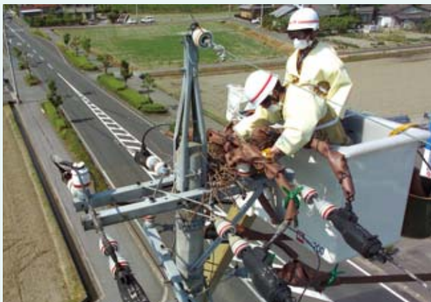
Crow's nest removal work
