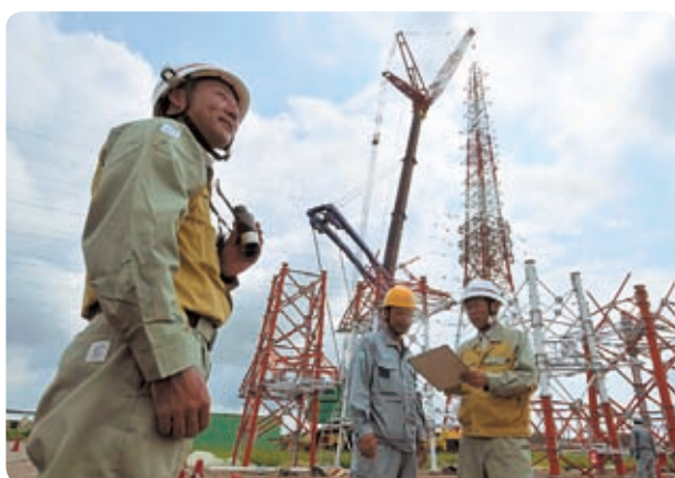
Work on power transmission lines to keep up with rising demand
