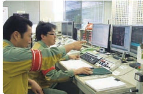
Remote operations with distribution line automation system
