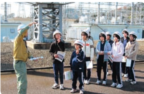
A tour of Tobu Substation (Toyota City, Aichi Prefecture)
