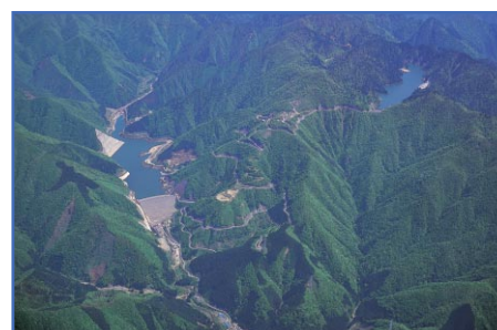
▲Okumino Hydroelectric Power Station
