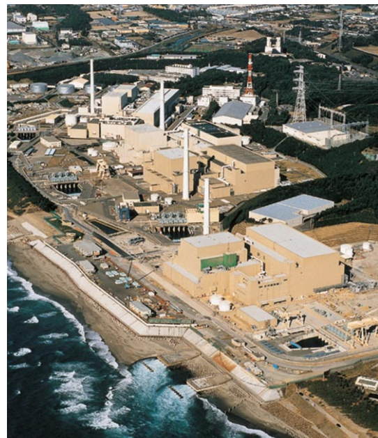
▲Hamaoka Nuclear Power Station
