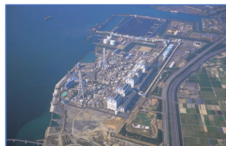
▲Hekinan Thermal Power Station
