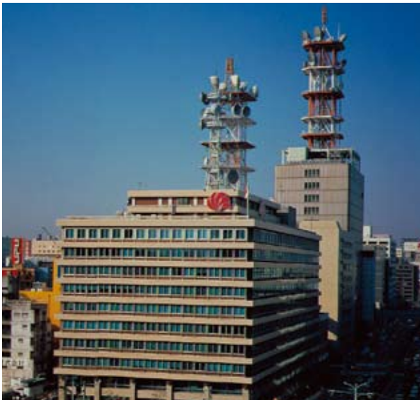
Chubu Electric Power Co., Inc. (head office)
