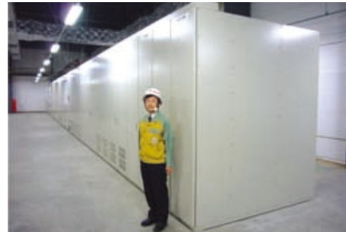
High Voltage Large Capacity Momentary Voltage Dip Compensator using EDLC (Electric Double-Layer Capacitors) (10,000kVA/second compensation)
