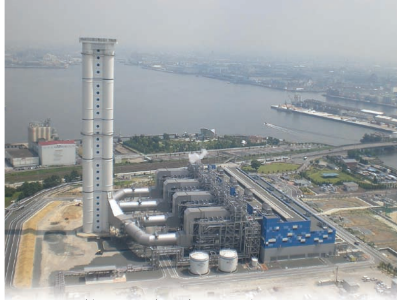
Shin-Nagoya Thermal Power Station Group No.8
