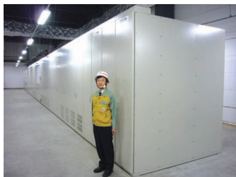
High Voltage Large Capacity Momentary Voltage Dip Compensator using EDLC (Electric Double-Layer Capacitors) (10,000 kVA/second compensation)
