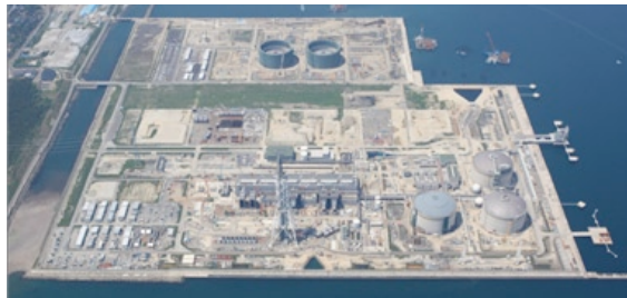
Joetsu Thermal Power Station (June 2011)
