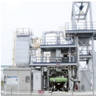
Stirling engine power generation facility that uses woody biomass
