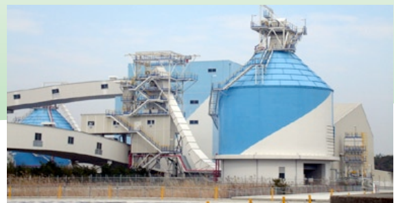
Biomass Fuel Facility (Hekinan Thermal Power Station)
