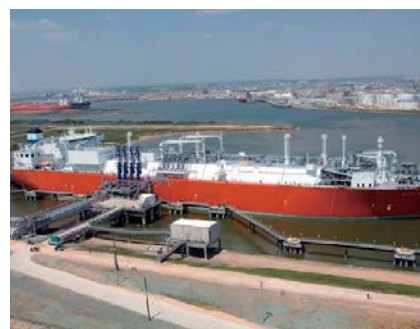
LNG carrier at the landing pier of the Freeport terminal
