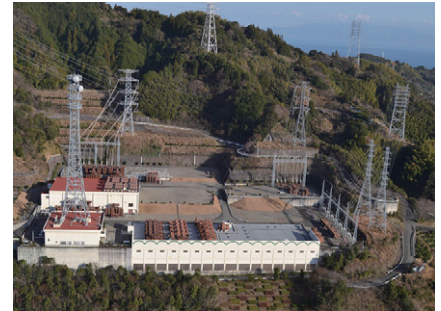
Higashi Shimizu Substation (Shizuoka City, Shizuoka Prefecture)
