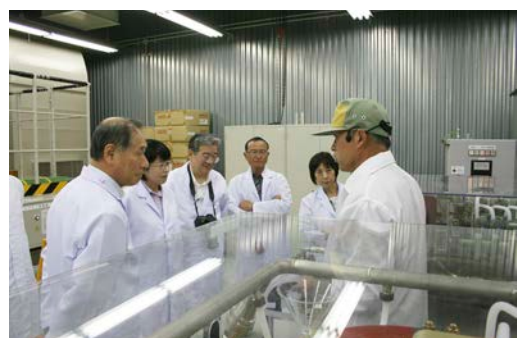
Committee members visiting the Higashi-Shimizu Substation (to see frequency converter systems)
