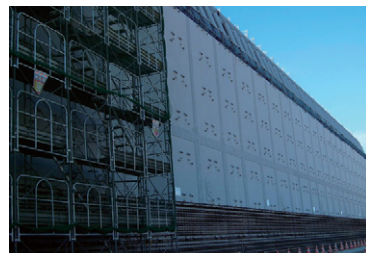
Breakwater (under construction)
