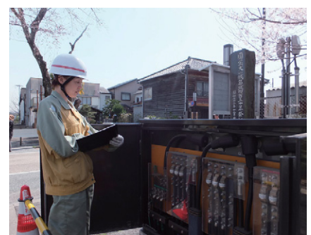
Inspection of the underground distribution equipment
