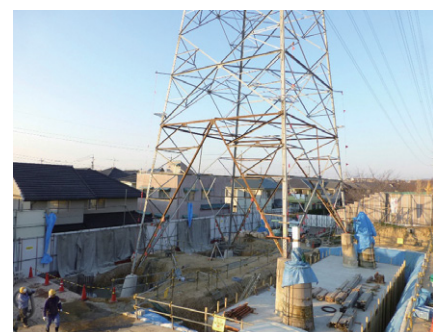
Groundwork in a residential area
