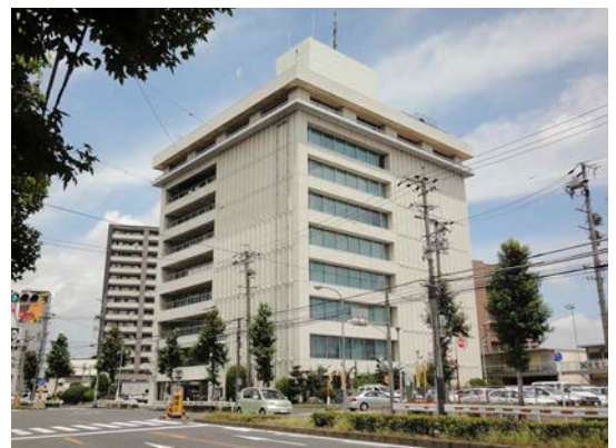
Renovated, energy-efficient, Atsuta Building (Atsuta-ku, Nagoya City)
