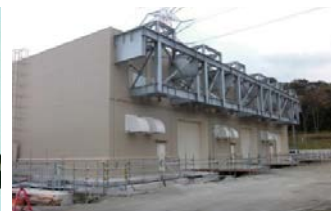
Building that houses the generator
