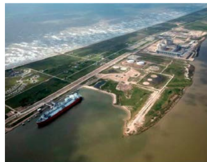
Full view of the Freeport terminal
