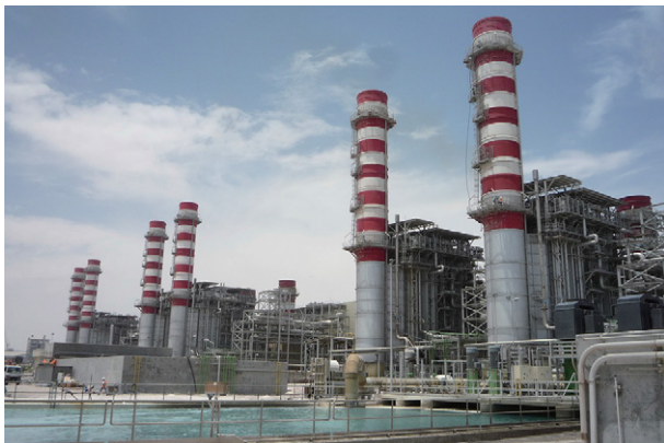
In Qatar, we have invested in a gas thermal power generation facility to build a multi-faceted relationship that is not limited to fuel procurement. (Gas thermal power generation project in Mesaieed, Qatar)
