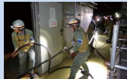
Cable installation exercise (done with the lights turned off)
