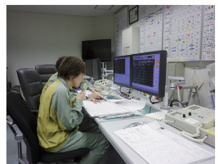
Issuing a distribution line switching order
