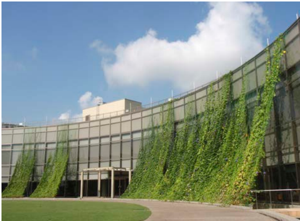
Green curtain developed at the East Plaza Ikomai Hall (Togo Town, Aichi County)
