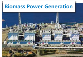
Biomass Power Generation Hekinan Thermal Power Station (Hekinan City, Aichi Prefecture) * Biomass-coal co-fired
