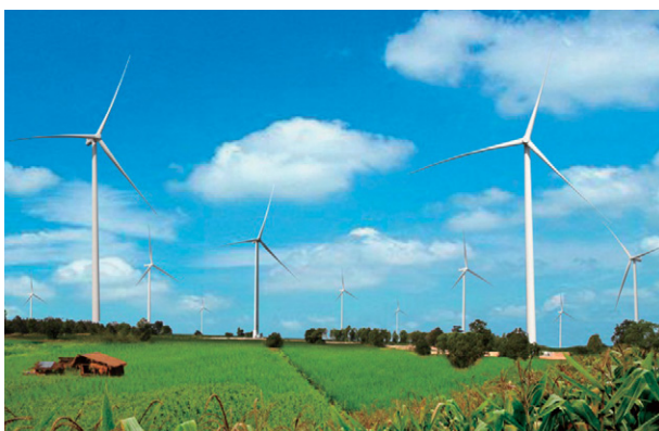
Southeast Asia's largest wind power generation project, in which Chubu Electric Power has invested (Nakhon Ratchasima Province, Thailand)
