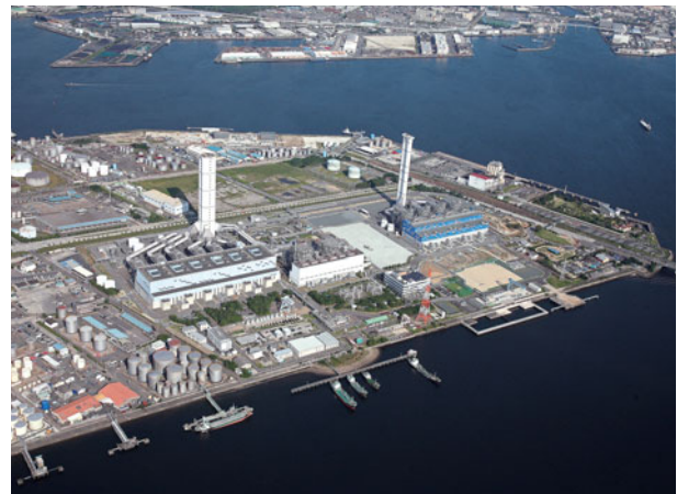
▲ Shin-Nagoya Thermal Power Station (in Shiomi-cho, Minato-ku, Nagoya City)
