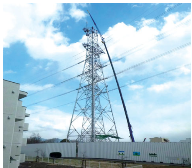
▲ Assembly of a transmission line tower
