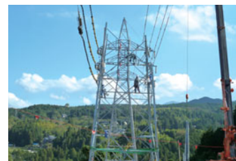
▲ Work on a transmission line tower
