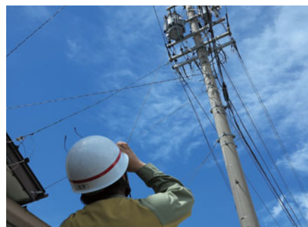
Patrolling the power distribution facilities
