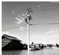
Restored distribution line after Typhoon Isewan (1959)
