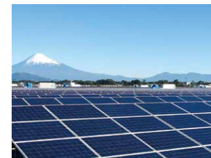
Mega Solar Shimizu (2015)
