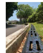
An example of the reuse of clearance metals
